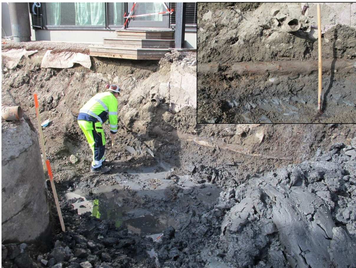
Figur 8: Trestokk in situ, under fundamenteringer for bygning.
